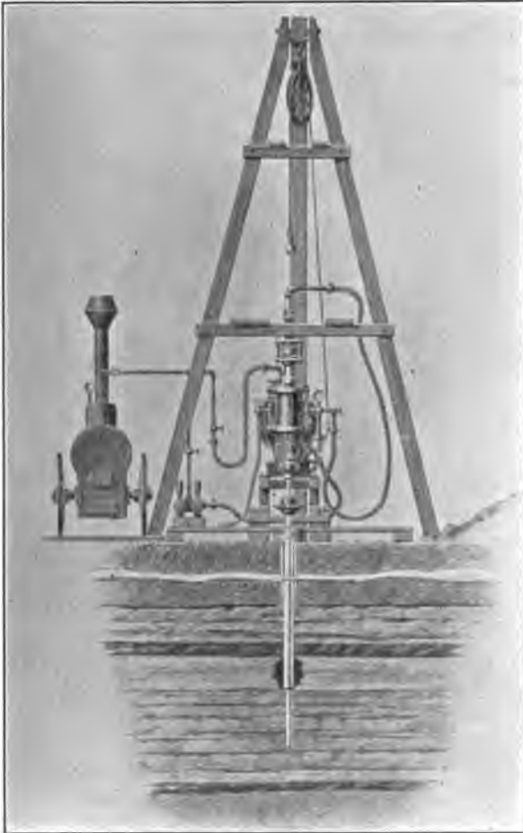
FIG. 8.—Arrangement of typical diamond drill outfit.
